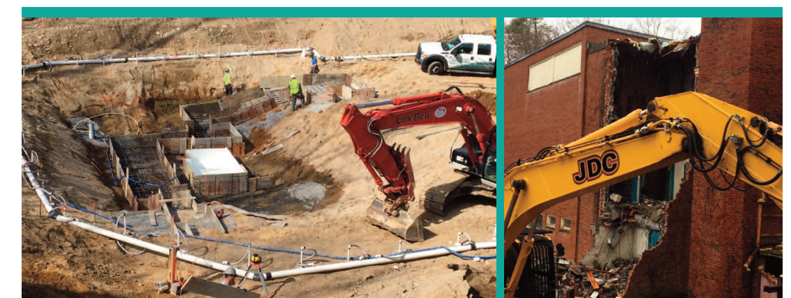
Demolition started in the spring of 2018 followed by excavation for the new wing. Construction is on schedule for a Grand Opening in Fall 2019.
